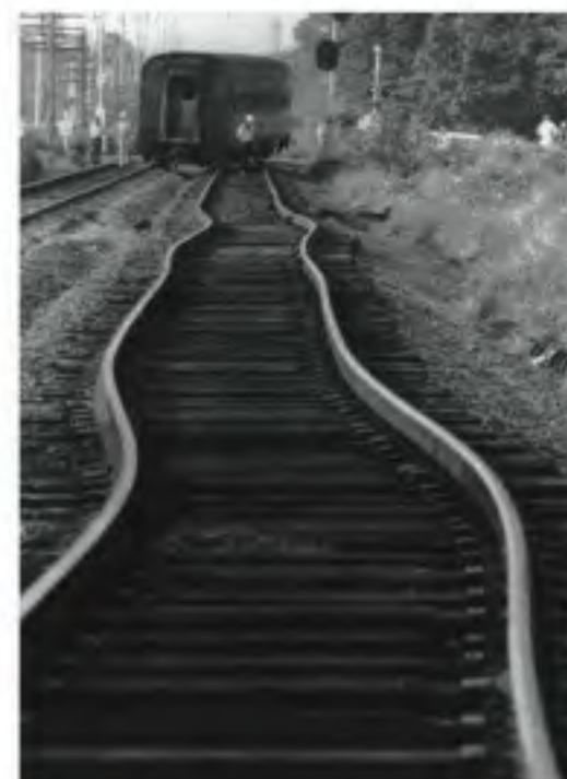
FIGURE 17.7 Thermal expansion distorted these tracks, causing a derailment. Expansion of long structures like this is best described using the coefficient of linear expansion.
