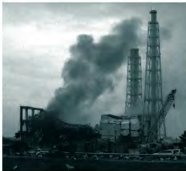
Smoke pours from a damaged reactor at Japan's Fukushima Dai-ichi nuclear power plant. How dependent is humankind on nuclear power?
