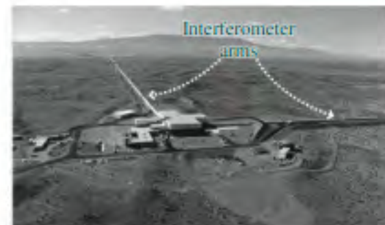
FIGURE 32.16 The LIGO instrument at Hanford, Washington, is an interferometer with 4-km arms. The light undergoes multiple reflections, giving an effective arm length of 300 km.
